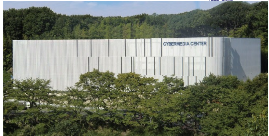
IT core as data center
