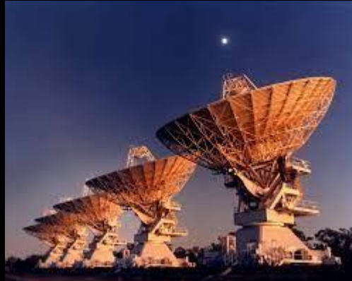
SKA Australia Telescope Facility
